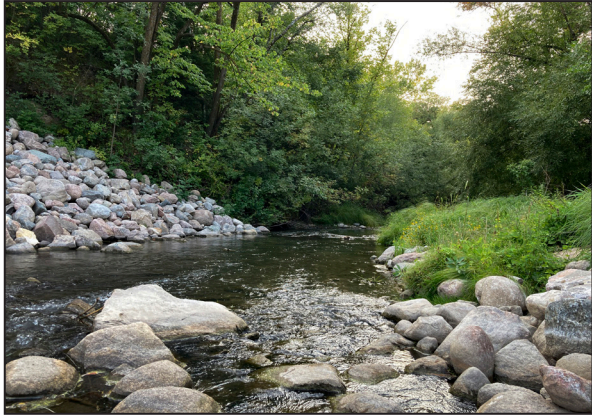
From top: Clean Water Fund-supported work on the Sand Hill River east of Beltrami stabilized head-cutting and allowed fish passage. Outdoor Heritage Fund-supported work removed a bridge and reconnected the floodplain. Photo Credits: Ann Wessel, BWSR
