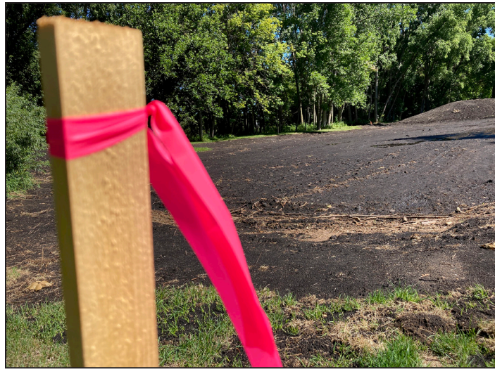
One day after a mid-August rain, a line of vegetative debris marked how high the water reached in the constructed wetland. The wetland, built on city-owned property bordering a ditch in Winsted, will filter about 15 acres of residential stormwater runoff bound for Winsted Lake. Photo Credit: Ann Wessel, BWSR
